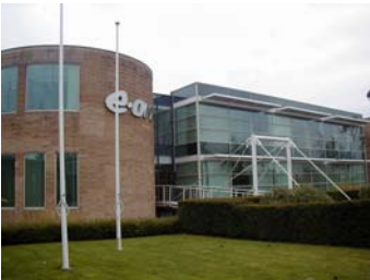
The Modern Main Entrance/Reception Building
