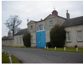
The Stables Building
